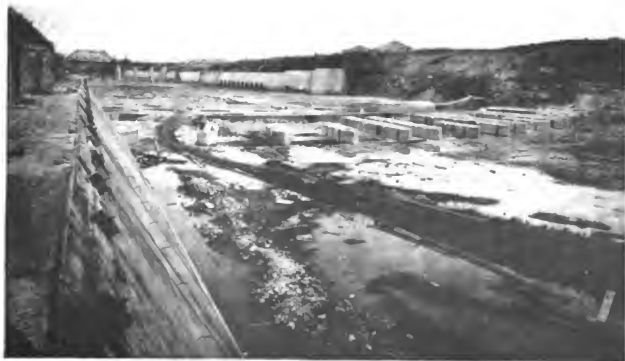
GATUN SPILLWAY LOOKING NORTH
